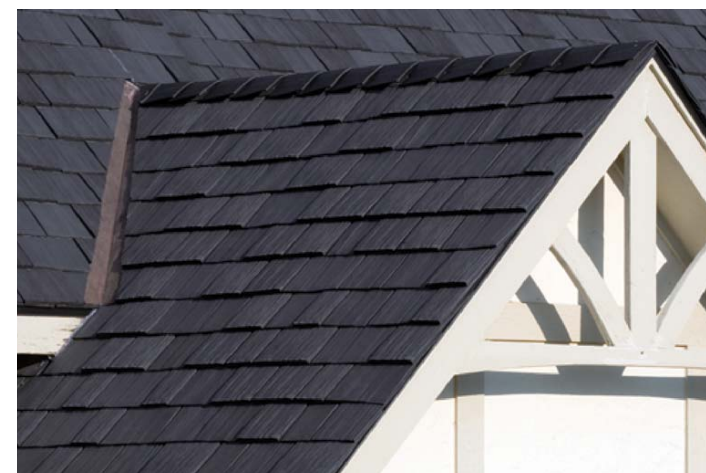
polymeric shake tile roof
