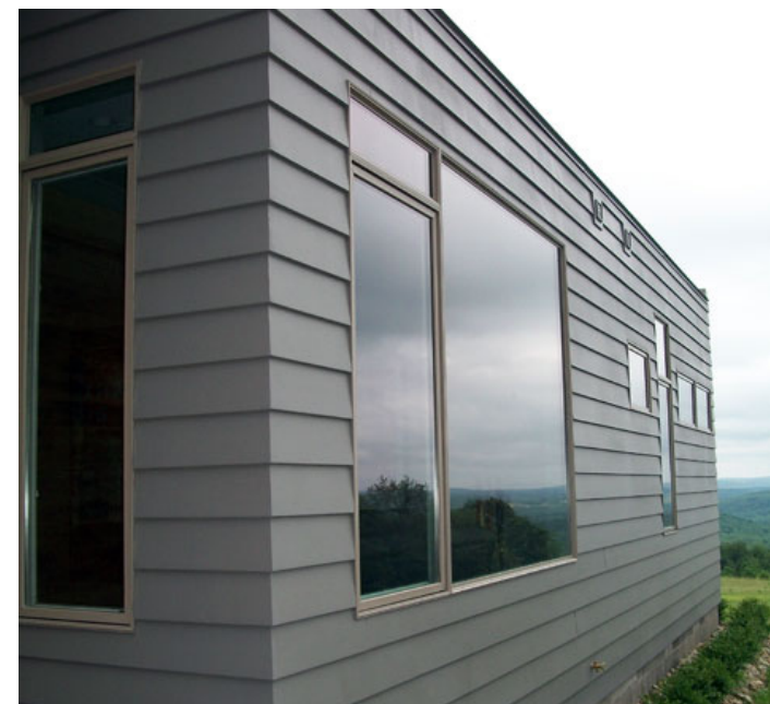
cementitious lap siding corner condition
